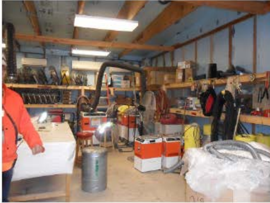
Temporary HVAC Shop
