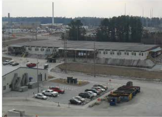
Construction Admin 54,000 sq. ft. (Temporary)
